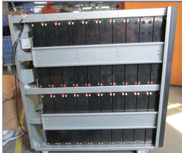
**notice:** while nstall the batteries the battery, please keep terminal away from metal case and the other terminal, avoid short circuit.
