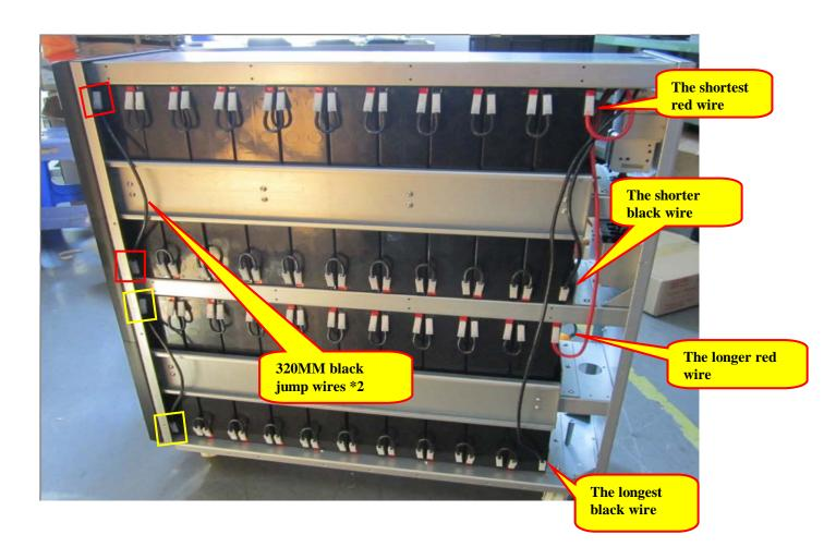
**notice:** make sure the position of the battery wires is right, the terminal should be inserted well.
